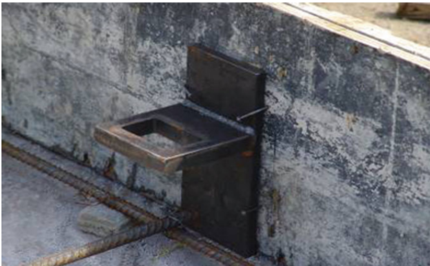
Fig. 3.19 Accelerometer mount cast in situ
