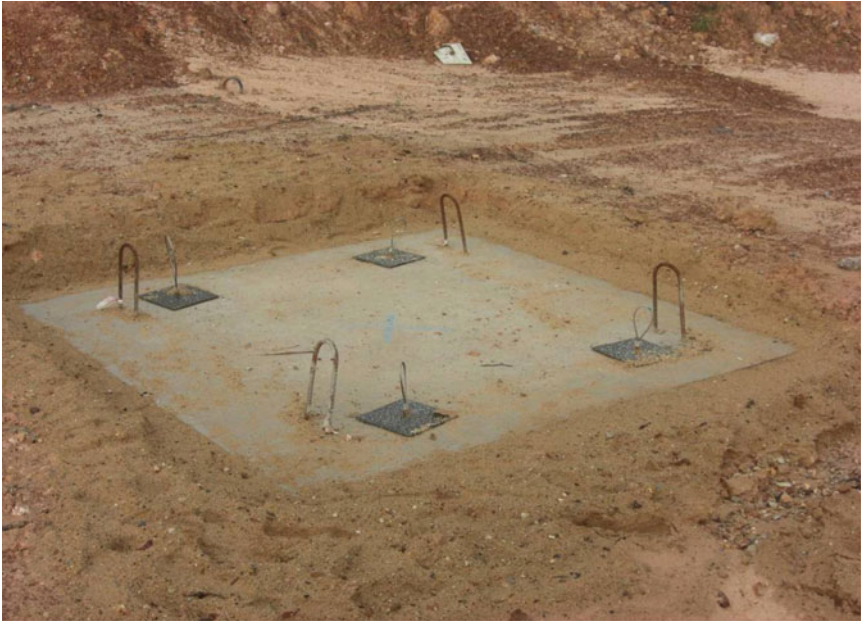
(a) Normal concrete pavement slab before blast event
