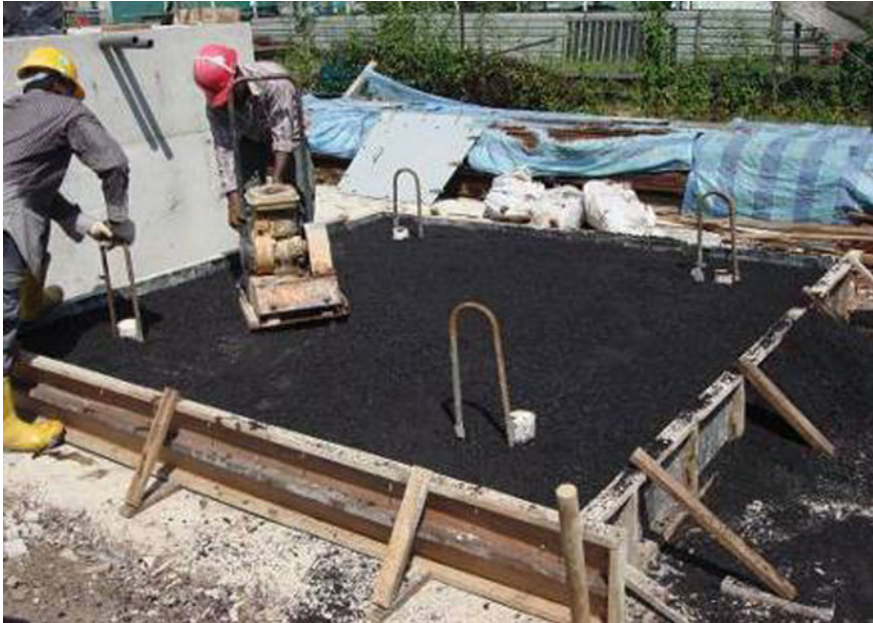
Fig. 3.6 Compaction of asphalt layer
