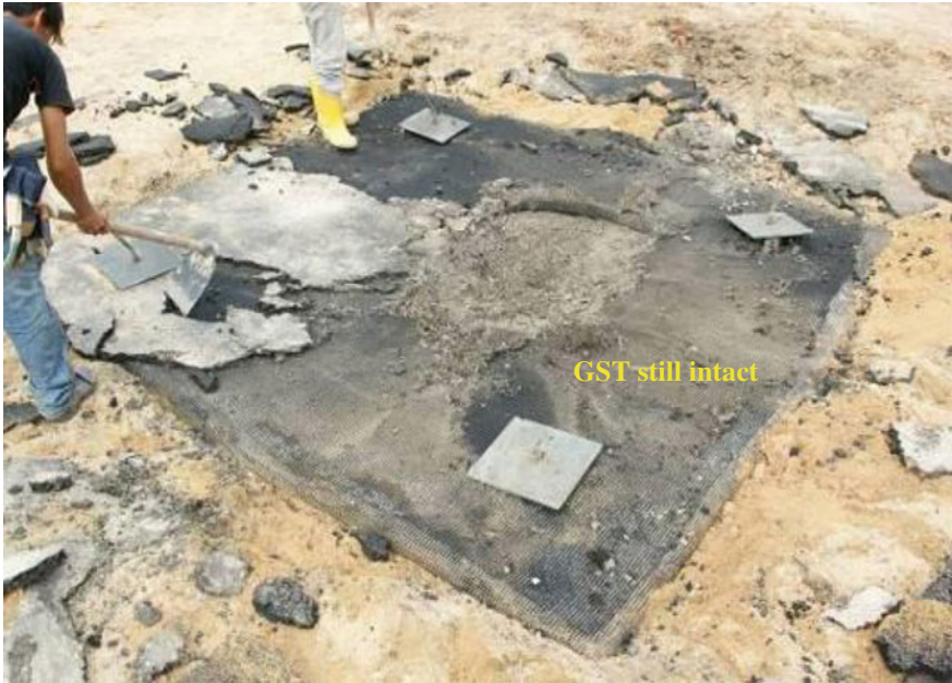
Fig. 3.36 Removal of top section of the AC layer for the Slab 2
