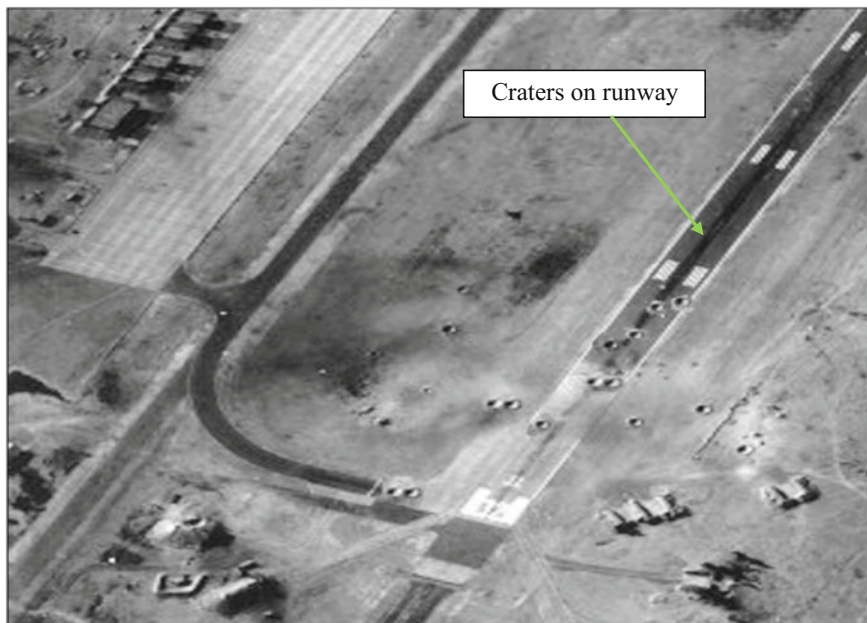
Fig. 1.1 The integrity of the runway was destroyed by blast and impact load. (after Chew et al. 2009)
