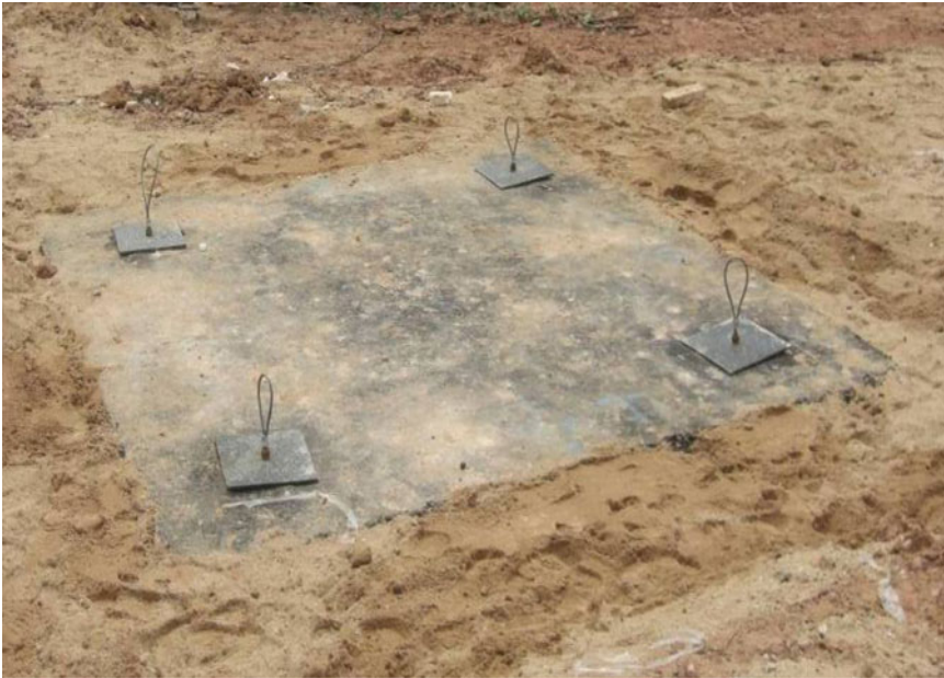
(b) Proposed new material pavement slab before blast event
