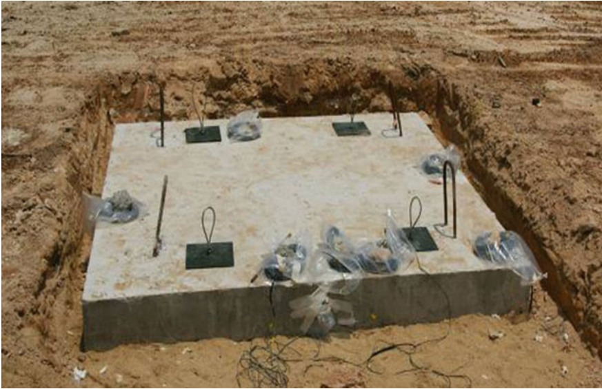
Fig. 3.11 Completed Slab 1 with anchoring at site
