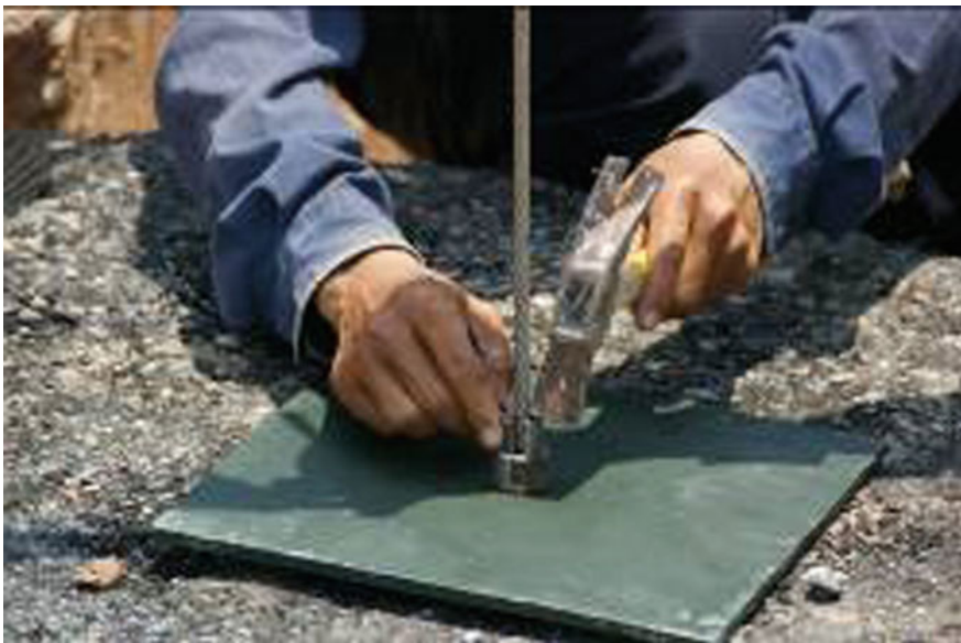
Fig. 3.10 Extraction of steel cable using excavator and anchoring of steel plates on surface of slab
