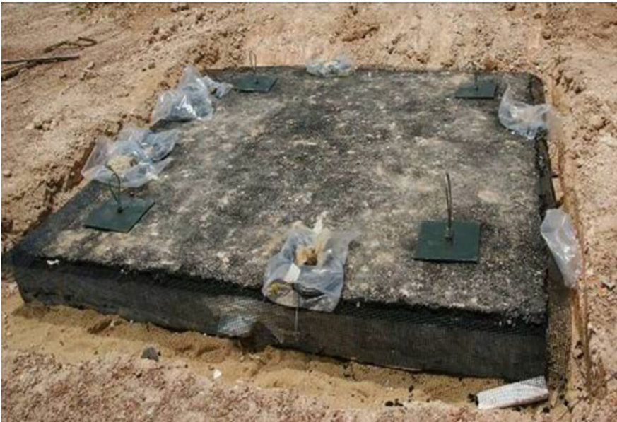
Fig. 3.12 Completed Slab 2 with Anchoring at site
